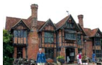
Above and left, Dorney Court; far left, the Savill Building at Windsor Great Park with its spectacular single-span roof made of green wood
