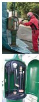
Above right, the petrol pump being shot-blasted; below, restored and re-painted
